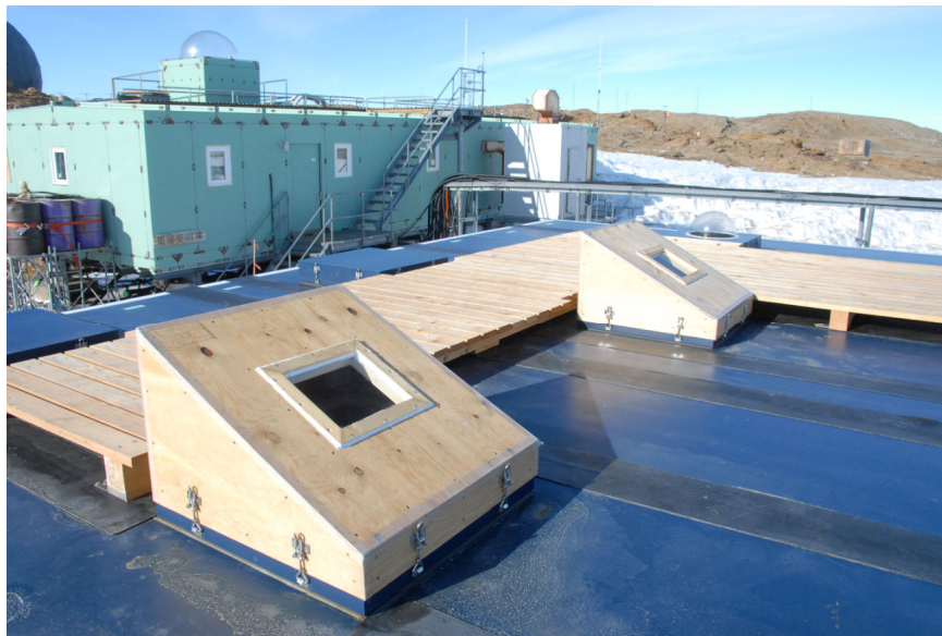
Figure 2-12. Skylight set on the roof of the optical building at Syowa Station. The window is tilted to direct the field of view of the spectrometer to the magnetic zenith.
