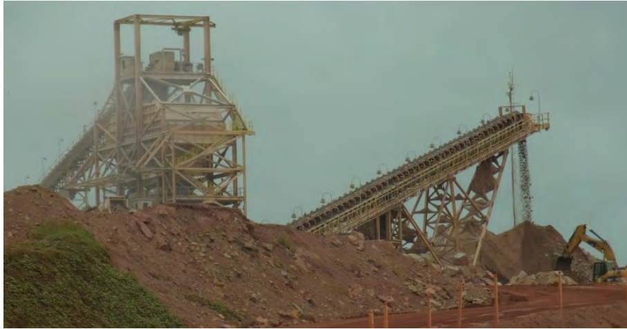
Fig. A.3: Crash ore plant.
