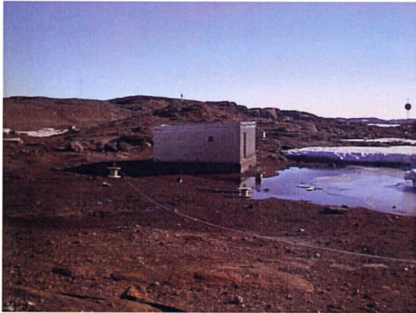
Figure 3.7 The seismograph room where Hydrogen maser frequency standards and associated devices are installed.
