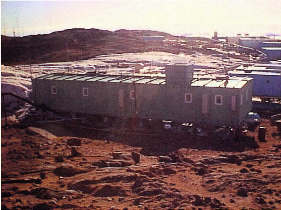
Figure 3.13 The satellite data reception room where the VLBI back-end system and the antenna pointing system are installed. The signals received by the 11m antenna are terminated in this room.
