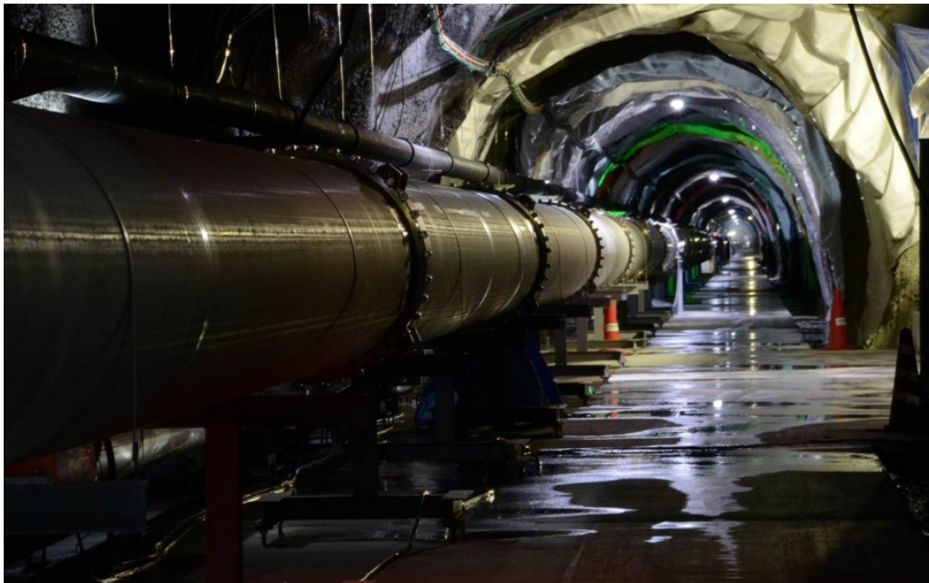
Figure 2.2: KAGRA is about 1000m underground, here it shows one of the 3km arms inside KAGRA tunnel
