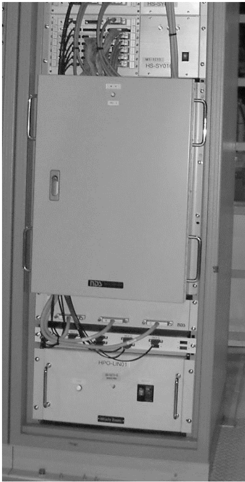
Fig. 3.20. Appearance of a new connector-box. Fig. (a) is a front view and Fig. (b) is a rear view of the new connector-box. The rear panel is used as a connector panel to attach signal cables from equipment.
